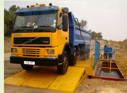
Portable closed-loop wheel washing systems for reducing onsite and offsite trackout during construction
